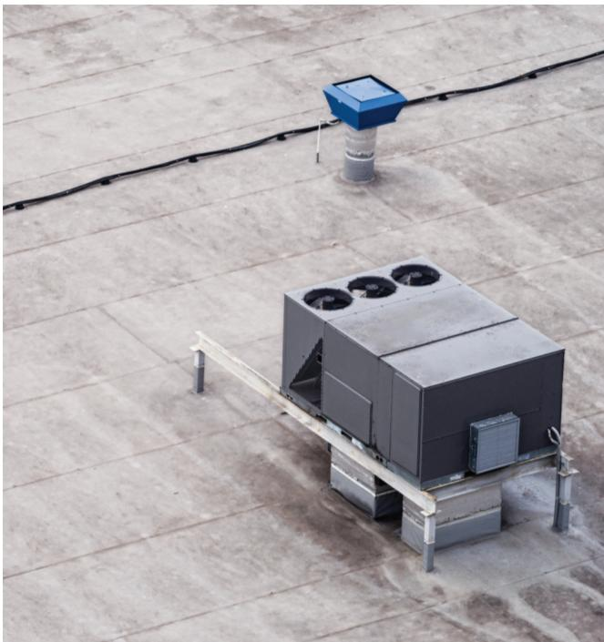
there are incentives for advanced rooftop controls (ARC). Supply fan controls account for more than 80 percent of ARC retrofit energy savings. ARC retrofits can reduce fan speeds up to 60 percent during the first stage of heating and cooling, and up to 40 percent when no heating or cooling is needed. ARC retrofits reduce supply fan speeds to pre-determined levels during heating, ventilating and air-conditioning modes.
