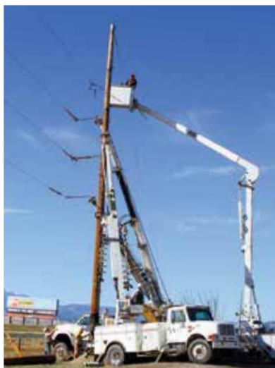
Line contractor replacing a transmission pole near Whitehall.
