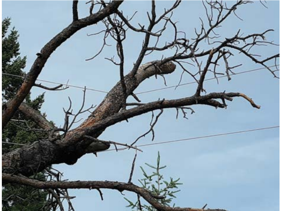
Downed trees and limbs can bring down power lines and they can hide electrical hazards. If you see a downed power line contact emergency services immediately. | PHOTO BY TOWNSEND FOREMAN JOHN MOOS
