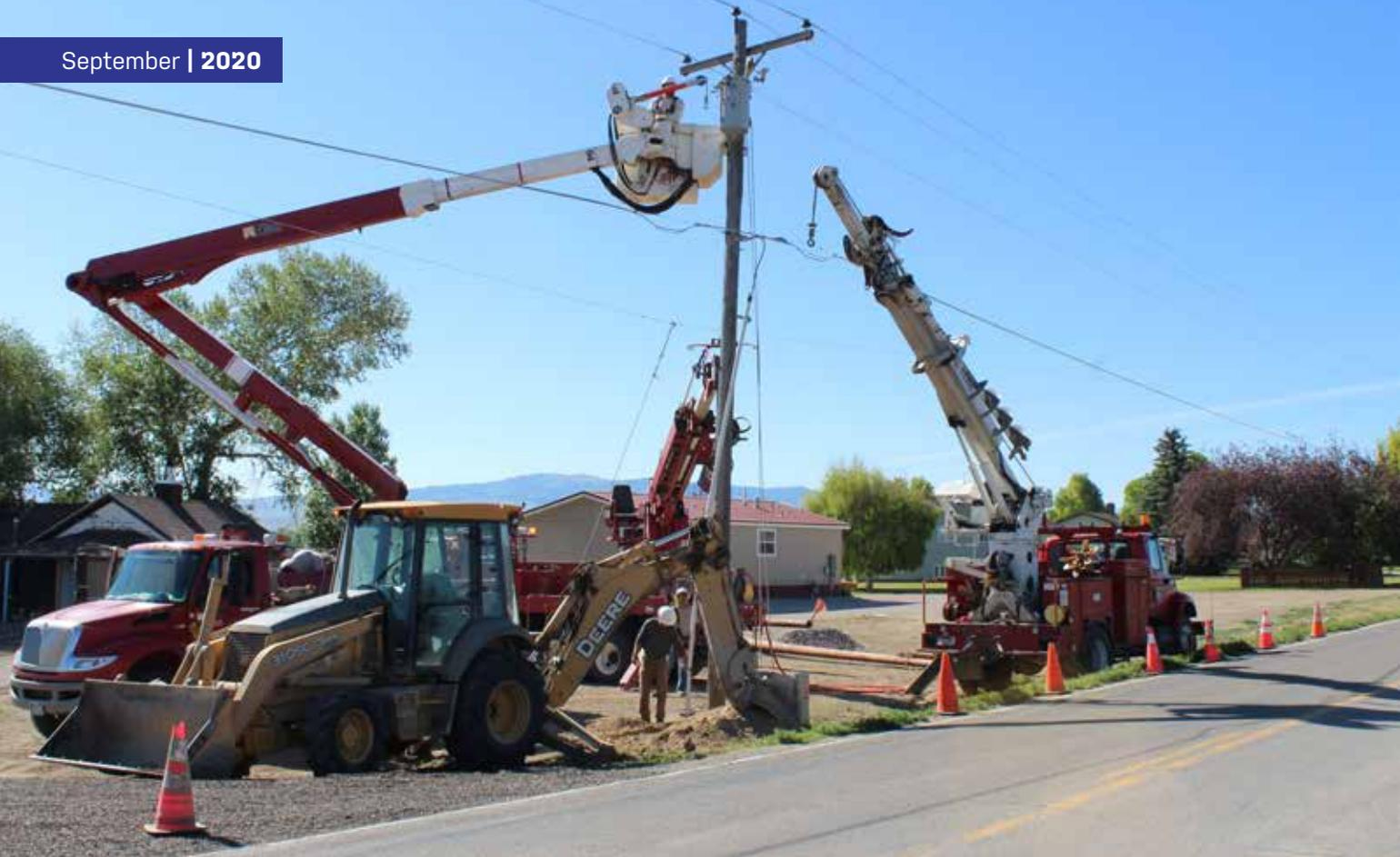
Pictured is Vigilante Electric Cooperative's line crew changing a pole north of Dillon. This pole change was done "hot," so the power was never interrupted to the members off this circuit. | PHOTO BY ROD SIRING
